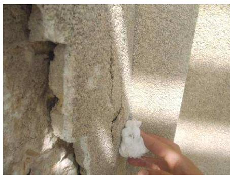
Fig. 2 – Detail of a zone with detachment.
