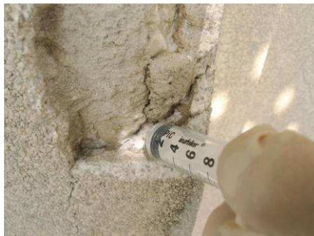
Fig. 8 - Grout application in building.
