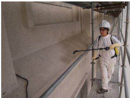
Fig. 7 – Lime water application in building
