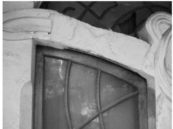
Figure 3. Scaling on calcareous stone
