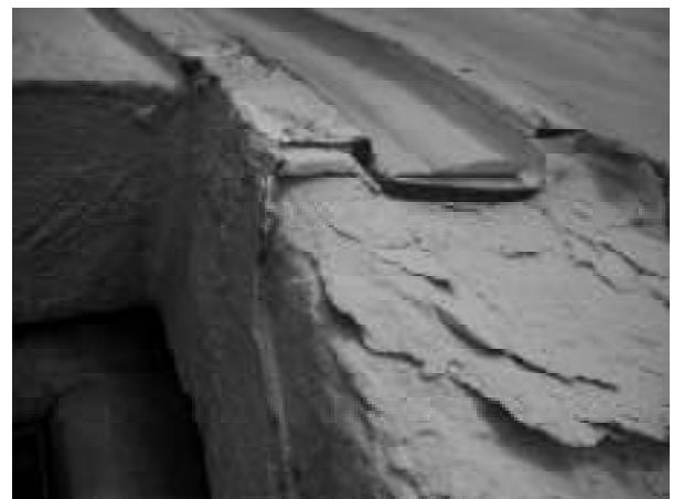
Figure 4. View of cement mortar layer between stone and lime mortar layer
